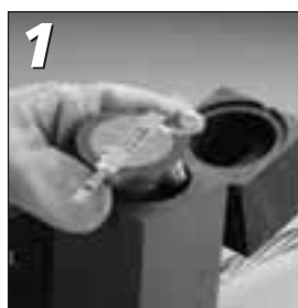
1 Insert CADWELD PLUS package into mould
